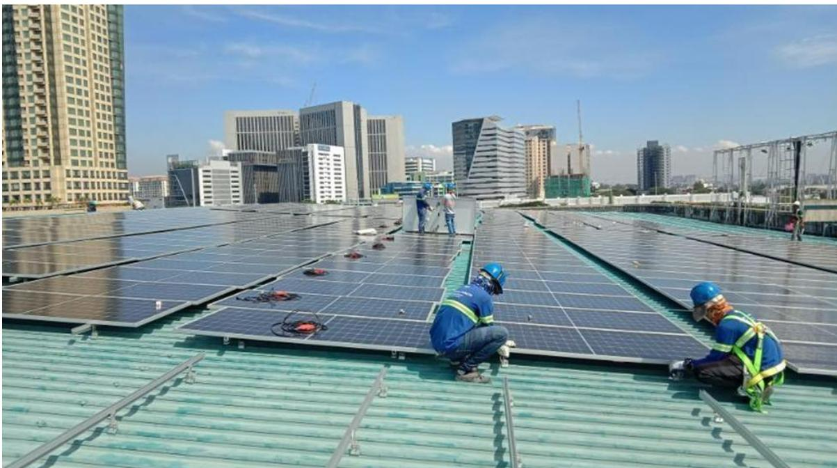
*Photo 2: Filinvest-ENGIE Renewable Energy Enterprise Inc workers installing photovoltaic solar panels on the Festival Mall rooftop*
